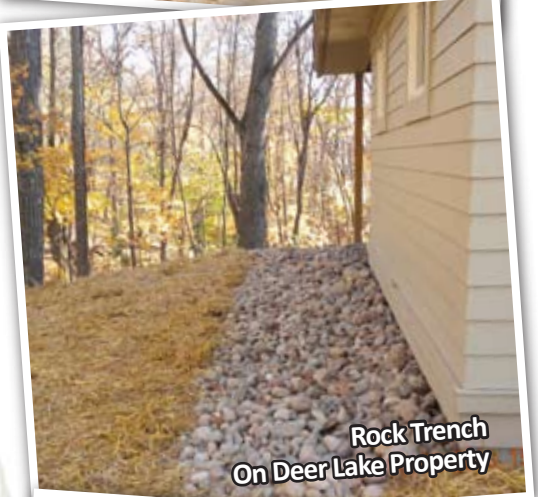
Rock Trench On Deer Lake Property
