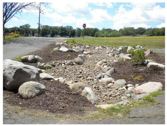
Figure 17. Balsam Lake Highway 46 Landing Rock Infiltration Pit
